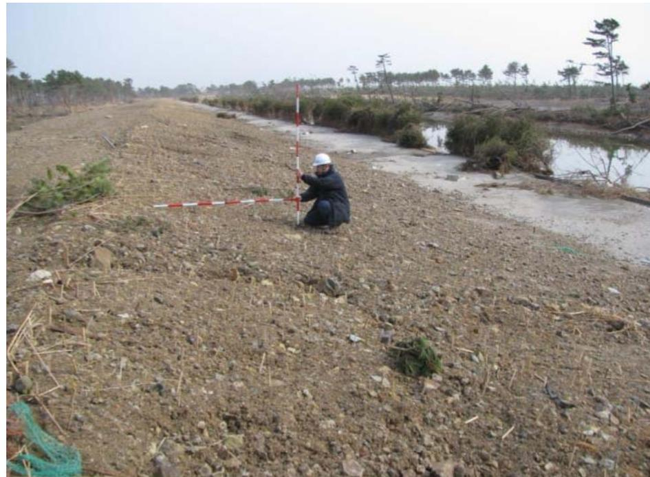
Combination of a severely damaged backside and a slightly damaged sea side was frequently observed for a trapezoidal dyke.
