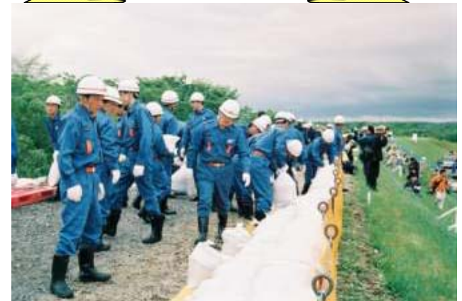
Deployment of sandbags
