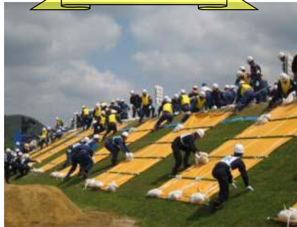
Protection of bank using plastic sheets
