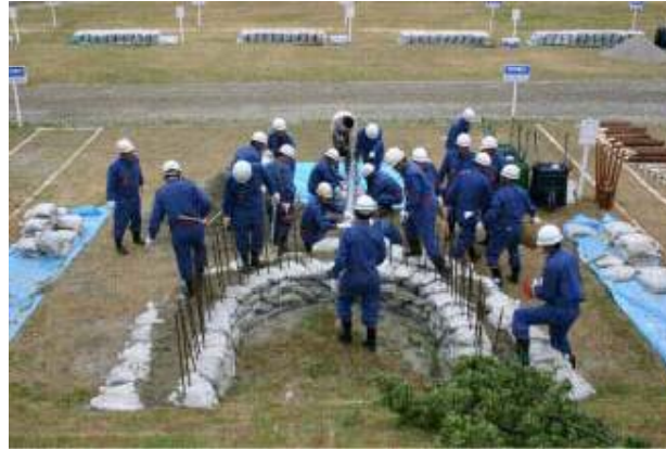
Circular sandbag loading work
